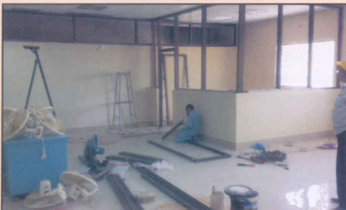
Rehabilitation is on full swing in Mechanical Engineering Department
