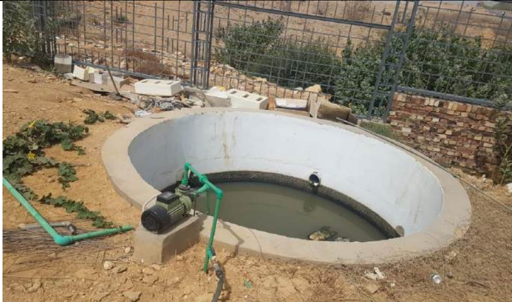
Soak pit, Mehran University of Engineering & Technology, Jamshoro.
