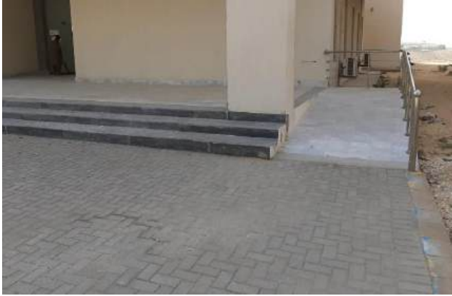
Ramp for Wheelchair at entrance of building (MUET, Jamshoro)
