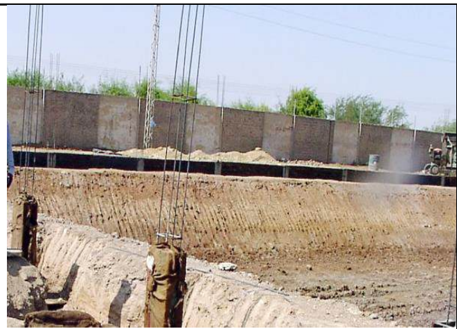
Jamashoro landfill site near thermal power station
