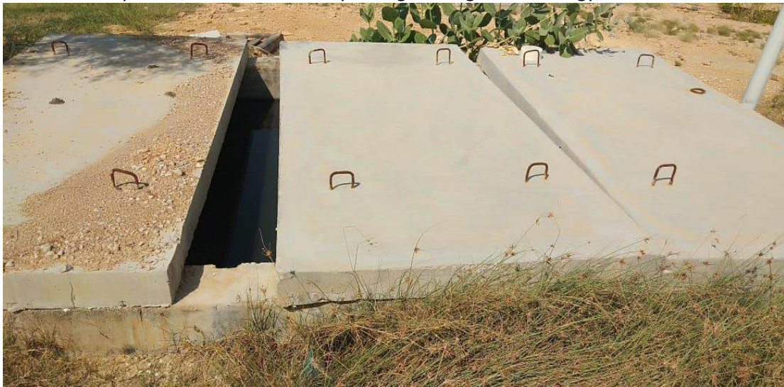
Sedimentation pit, Mehran University of Engineering & Technology, Jamshoro
